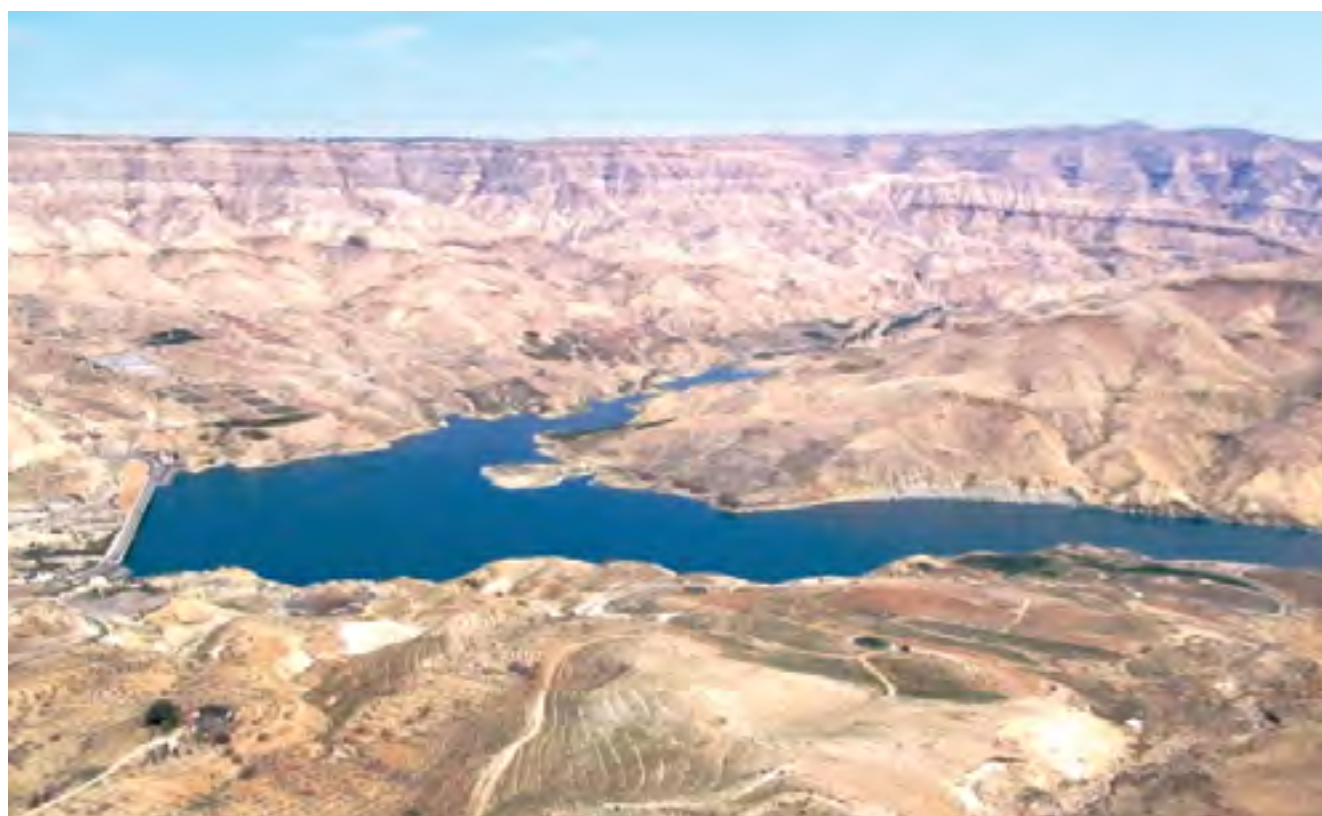
Figure 1-1 Mujib Dam 95km south of Amman with a capacity of 32 MCM
