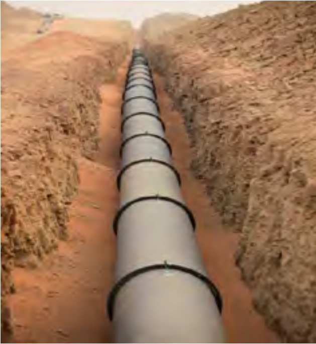
Figure 2-7 Security and Burial of Disi – Amman main pipelines
