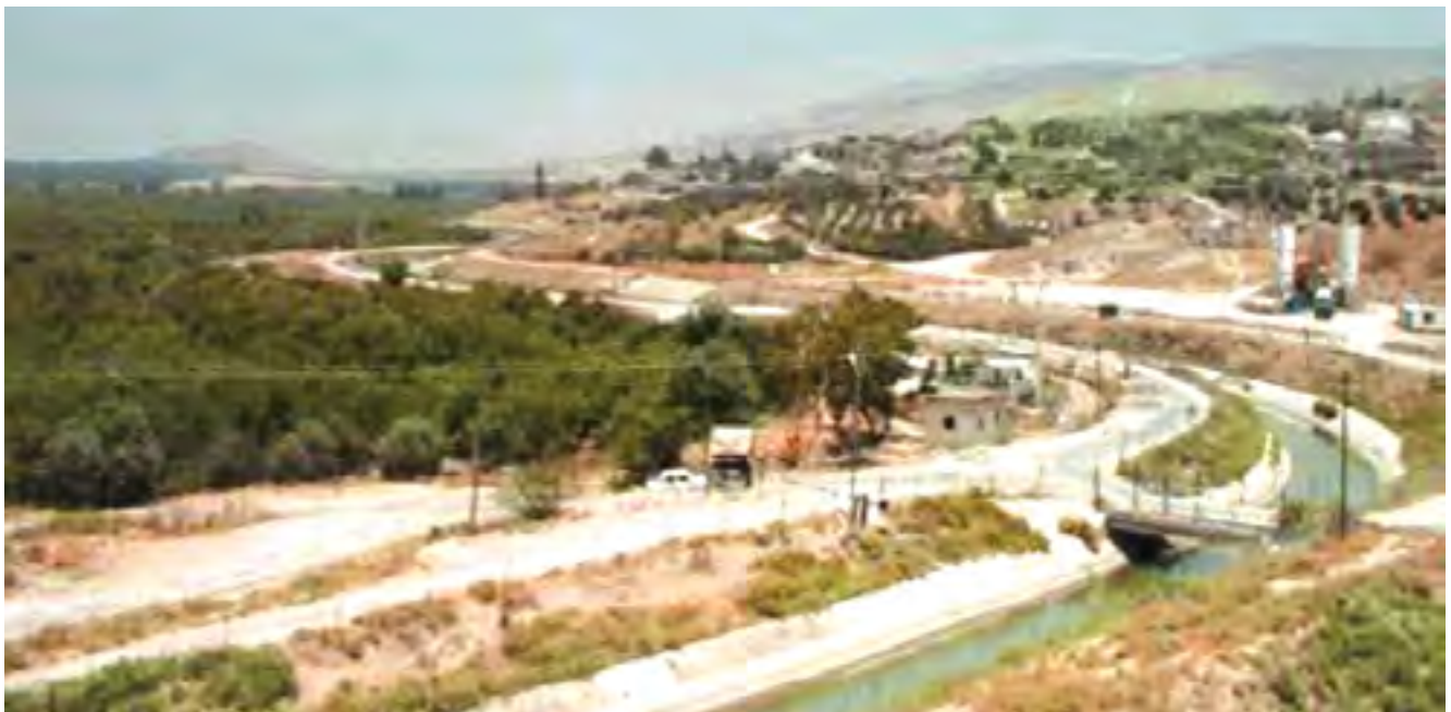
Figure 2-6 The KAC with security systems (Fences and cameras)
