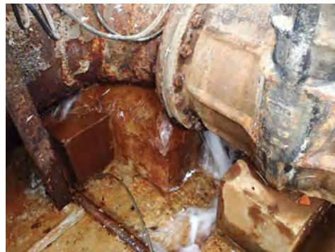
[Leakage at the Valve and joint in Pump Station]
