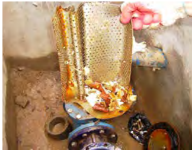
[Debris at Strainer or Rotating Part]
