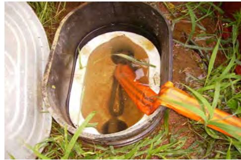
[An Illegal By-pass for Irrigation]
