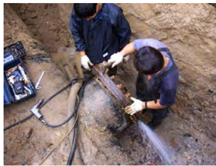
[Leakage at the Flange End Cap]
