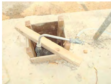
[An Illegal By-pass for Construction]
