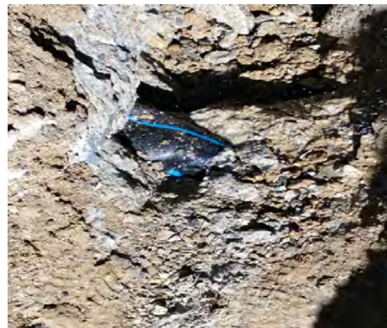
[Damage Caused by Casting Concrete above the Pipe]
