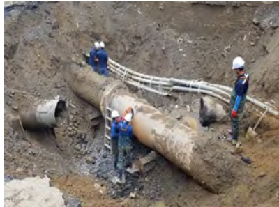
[Pipe Burst Caused by Poor Material DCIP and Stress Concentration]
