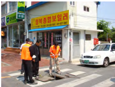
[Preparation for the Test: Boundary Valve Check and Closure]
