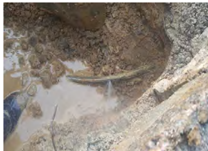
[Leakage in the Aged Pipe #1]
