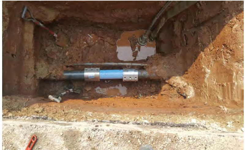
[Pipe Repair Using Repair Clamp #1]
