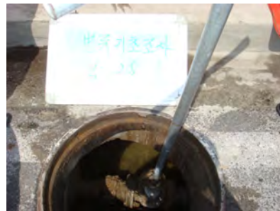
[Preparation for the Test: Boundary Valve Check and Closure]
