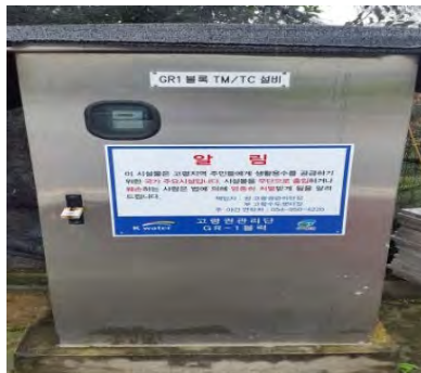
[Equipment for Monitoring and Control at DMA Inlet]
