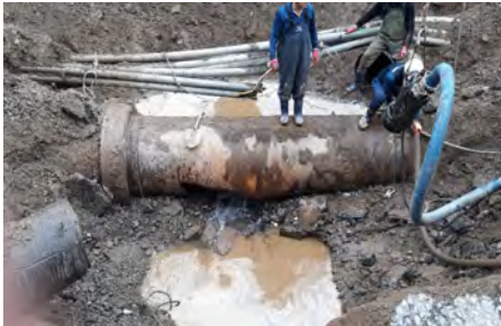
[Pipe Burst Caused by Poor Material DCIP and Stress Concentration]
