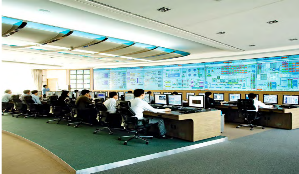
[Integrated Bulk Water Supply Monitoring System]
