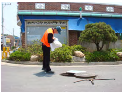
[Preparation for the Test: Boundary Valve Check and Closure]
