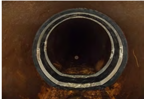
[Leakage Repair Using Backing Band]
