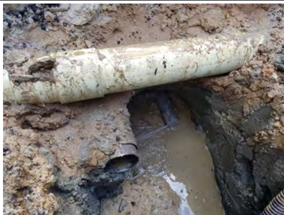
[Leakage Caused by Bad Finish]
