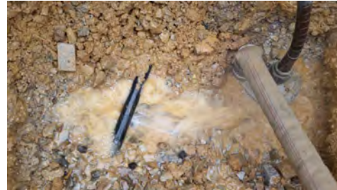
[Leaks Caused By Inappropriate Bedding]
