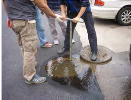
[Closing the Leaking Valve]
