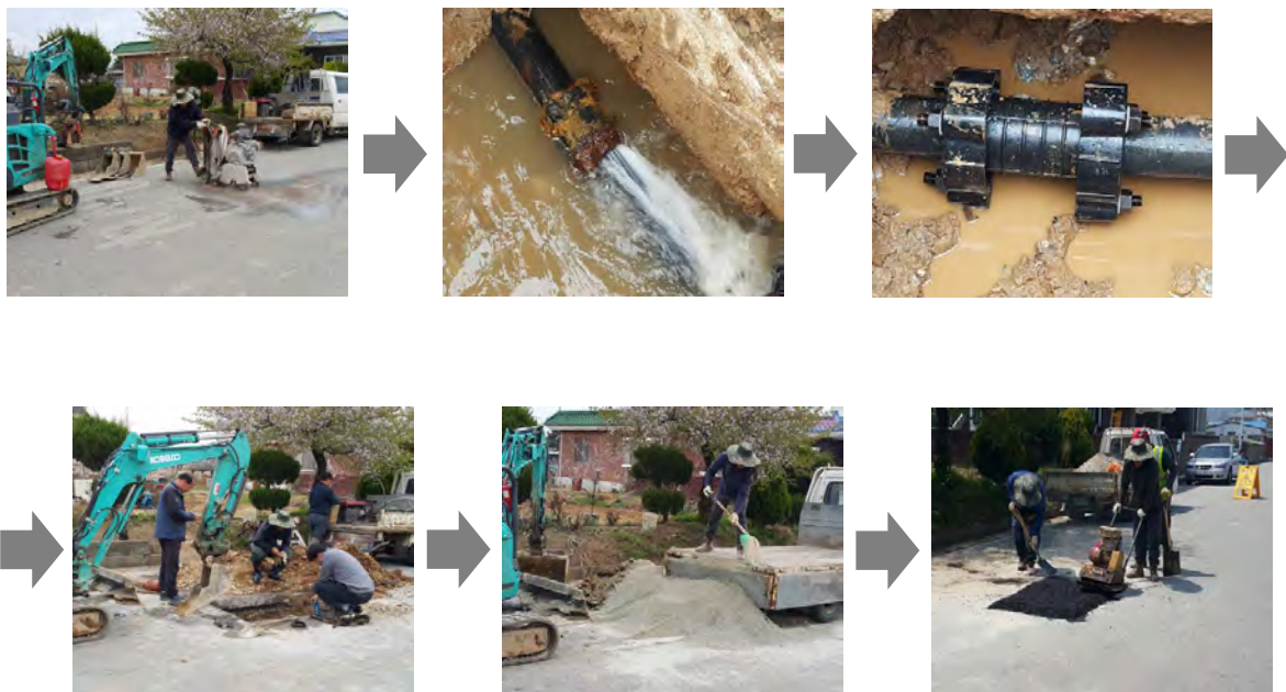
[Open Trench Replacement - Fittings, PE D100 mm]
