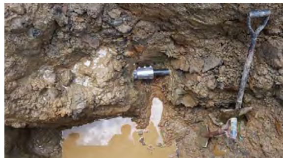
[Pipe Repair Using Repair Clamp #2]
