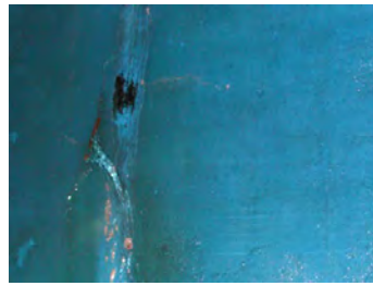
[Delamination and Leakage at Distribution Reservoir Wall]
