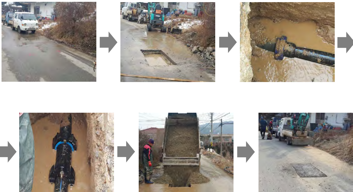
[Open Trench Replacement - Fittings, PE D100 mm]
