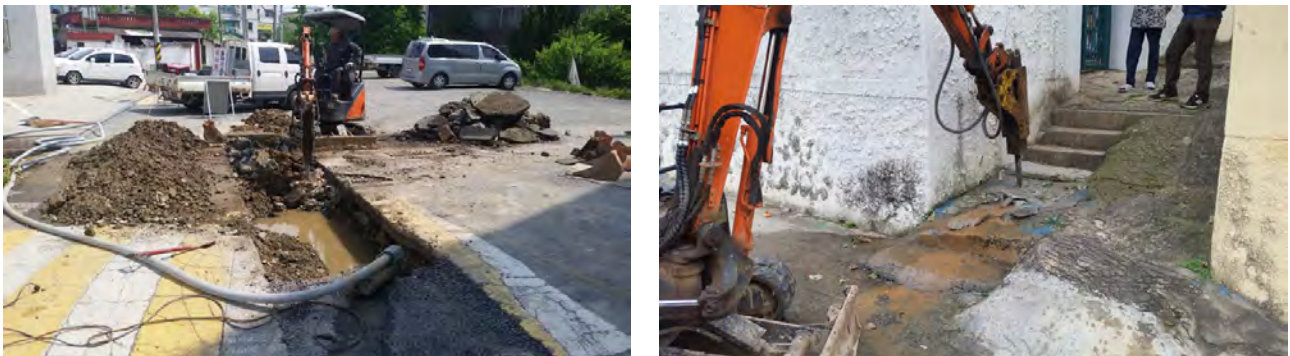
[Open Trench Method]
