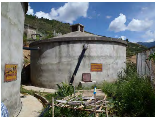
[Overflow at Distribution Reservoir]
