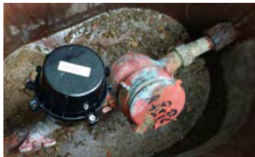
[Installing a Noise Logger on a Valve or Meter]
