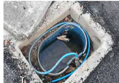
[Leakage at the Meter Box]
