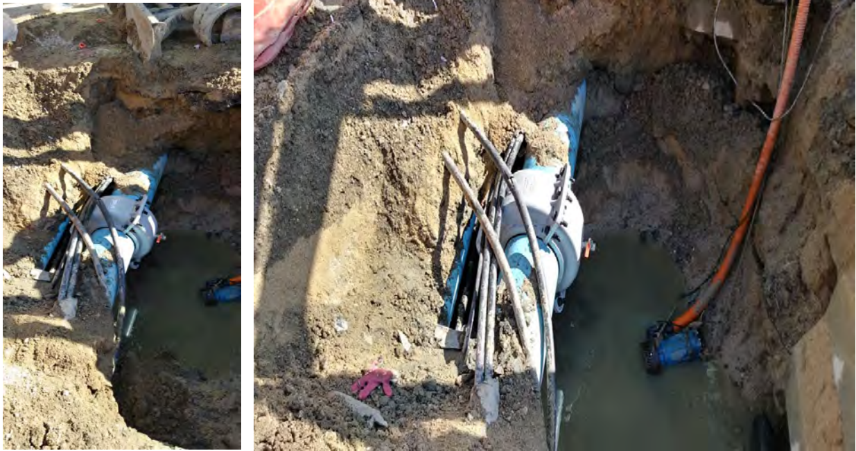
[Pipe Repair Using a Mechanical Joint (확인필요)]
