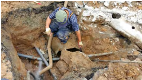
[Leaks Caused By Inappropriate Bedding]
