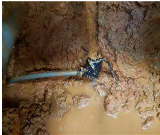
[Improper Repair Using Tape]
