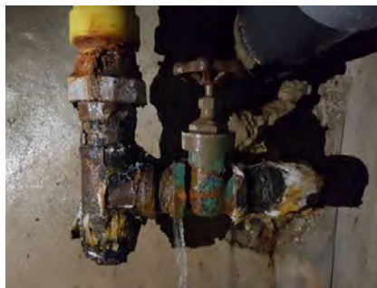
[Leakage at the Aged Valve #1]
