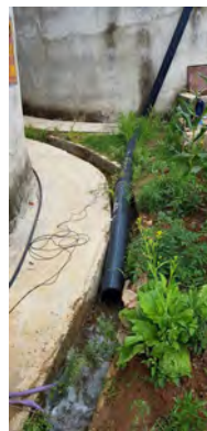
[Overflow at Distribution Reservoir]
