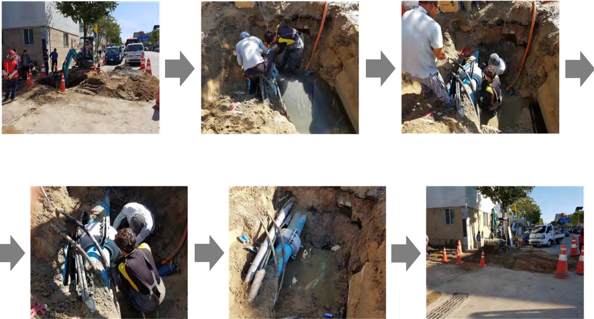
[Open Trench Replacement - Fittings, SP D300 mm]
