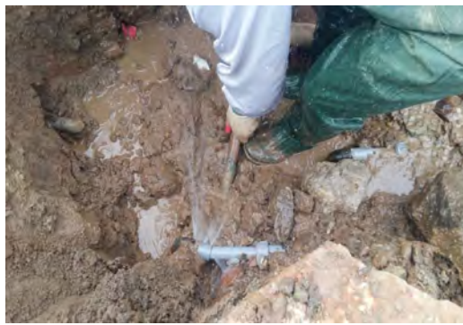
[Leakage Caused by Excessive Joint Deflection]
