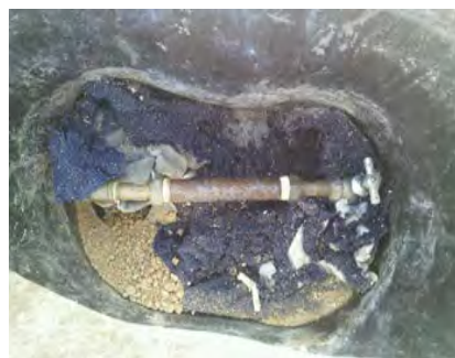
[An Illegal By-pass at a Water Meter]
