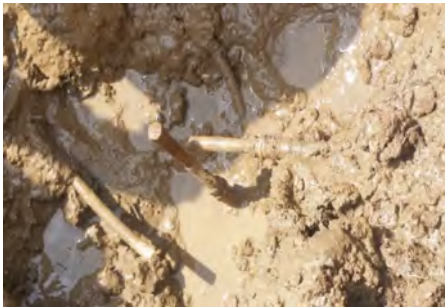
[Improper Repair Using a Wooden Needle]
