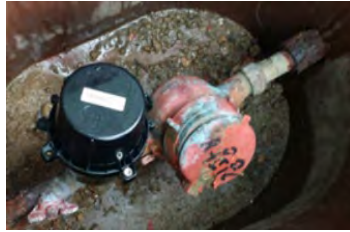
[Installing a Noise Logger on a Valve or Meter]
