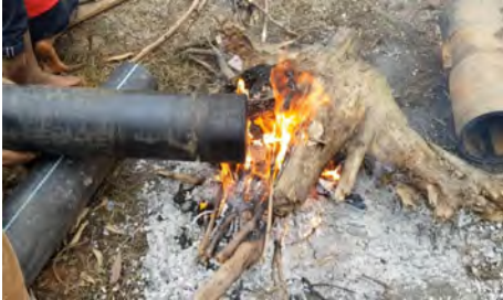
[Improper Joint Connection]
